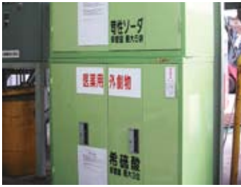
Storage of toxic substances at Kyoto Machinery Plant
