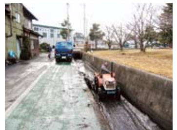
Waterway clean-up at Shiga Plant (January 28, 2006)
