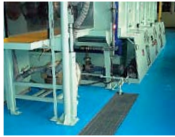
Installation of emergency drainage facilities at Kyoto Electronic Plant
